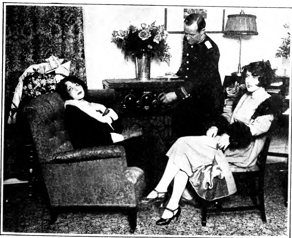
RADIO EQUIPMENT FOR THE HOTEL
